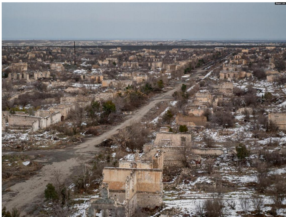
Fig 5. Completely destroyed Aghdam city after Armenian occupation.
